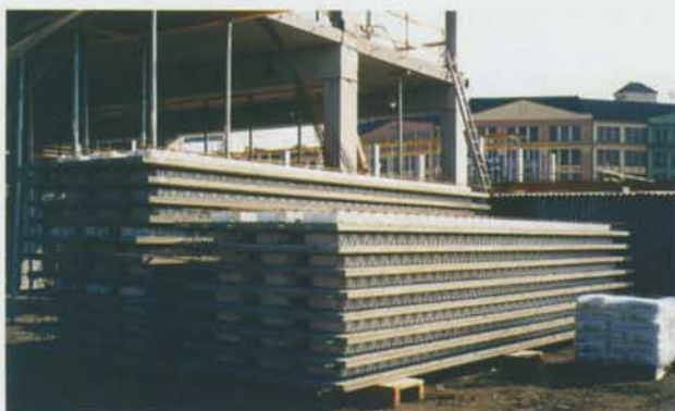
Fig. 7 Filigrane slabs with lightweight polystyrene belts
